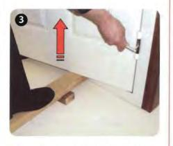
Lift and support the door to the required height whilst securing the socket screws. Replace the covers.
