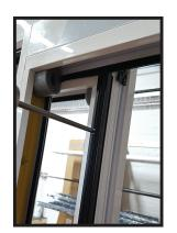
Re-fit the plastic interlock screws – these pick up on the back of the cover trim and secure it in place
