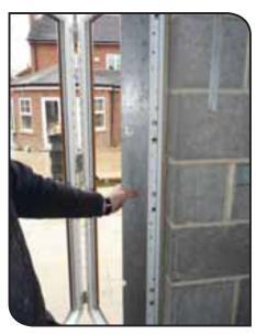
The frame head should then be fixed ensuring that it is parallel with the cill, again without twist and distortion. This can be aided by the use of a timber 'lat' or similar, cut to the internal height of the frame rebate and positioned along the width as a guide whilst fixing the head
