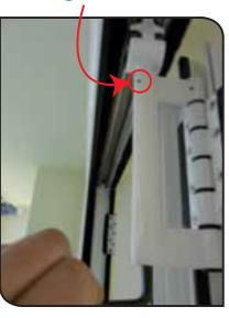
Commence glazing starting with the first hinged door onto the frame. Each unit should be 'toe and heeled'.
