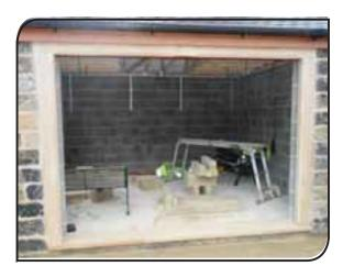
Suitable fixings should be used to secure the frame positioning 150mm to 250mm from each corner, then at a maximum of 600mm centers thereafter. Adequate support should be positioned between the brickwork and frame to prevent distortion when tightening the fixings.
