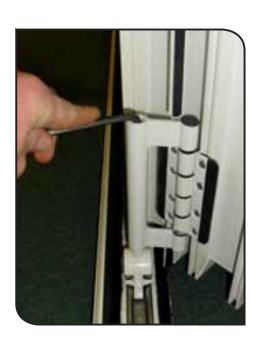
1 0. Top rollers should be adjusted to maintain compression/contact against the track.
