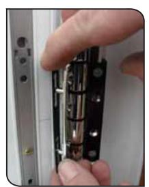
13. Compression adjustment can be made by rotating the cap at the end of the shoot bolts. Loosen the locking screw first then lock off once adjusted
