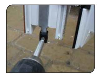
14. Any final adjustment then can be made to the wheel position then lock off the grub screw
