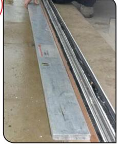
Silicone sealant should be applied to the drilled holes on the frame cill before the fixings are inserted to prevent water seepage.
