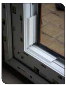
We strongly advise the use of our glazing platforms as illustrated above. 12. The nominal gap between the doors is 8mm. This can be adjusted to a minimum of 6mm and a maximum of 10mm by adding or removing the 1mm shim packers at each hinge point. The hinges have to be unscrewed in order to do this.
